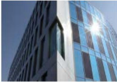
Figure 4. BIPV Solar Cells as Glazing Facades<sup>9</sup>
