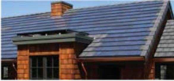
Figure 3. BIPV as Roof Tiles<sup>8</sup>
